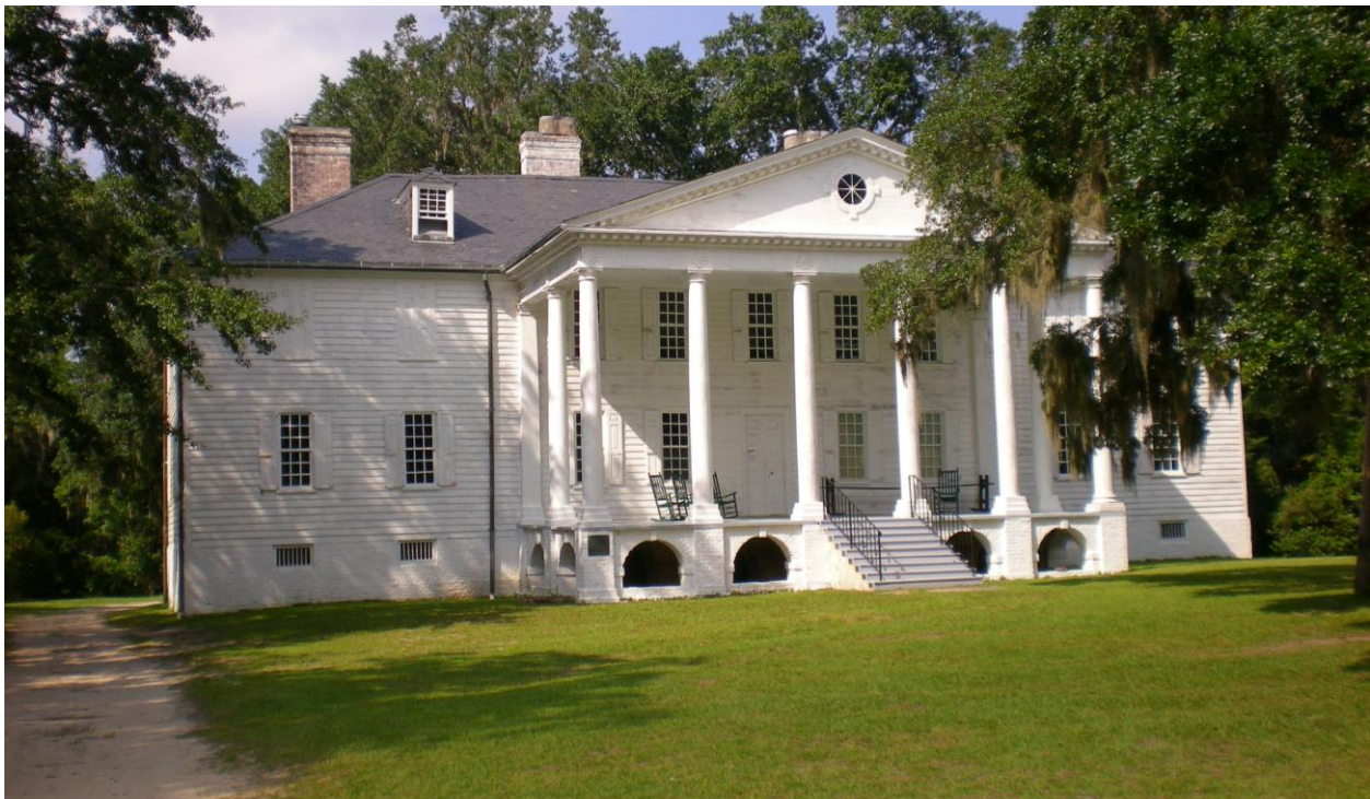
Figure 1 - Hampton Plantation [late eighteenth century], South Carolina
